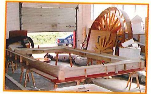
View into our manufacturing-plant
