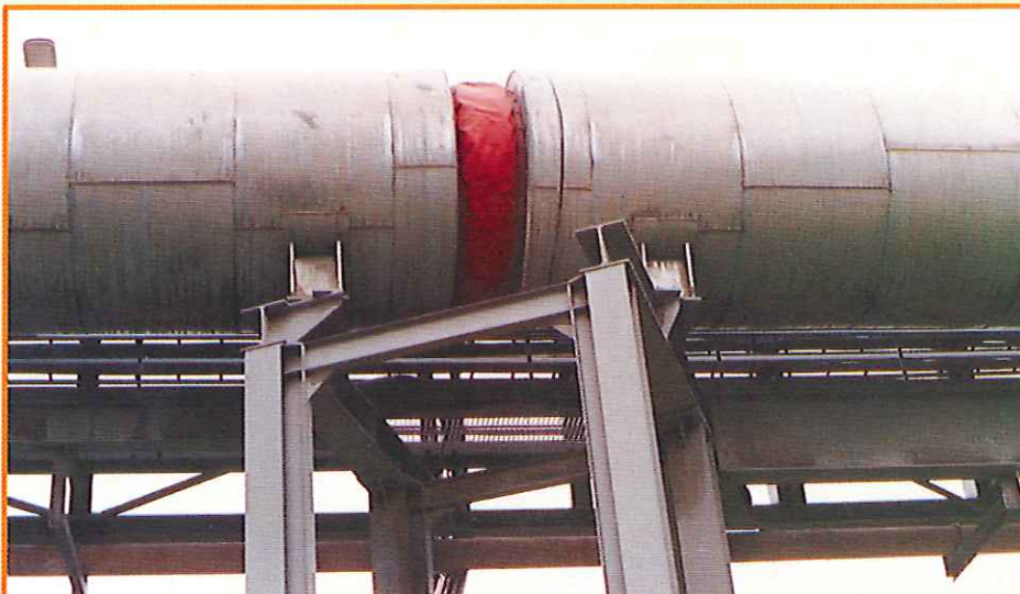
Flue gas recirculation in a cement plant.
