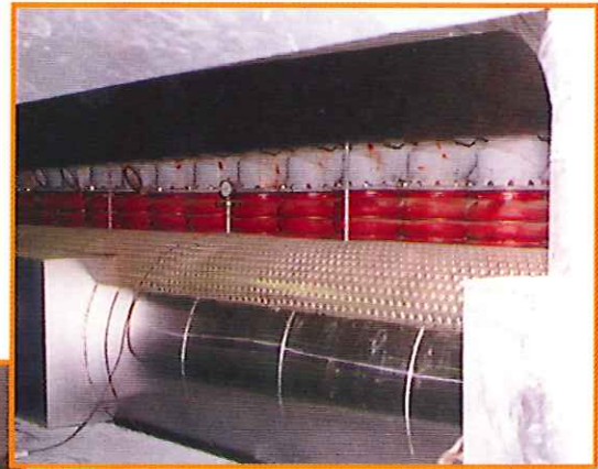
Incinerator plants - flue gas-recirculation / jet pipes
