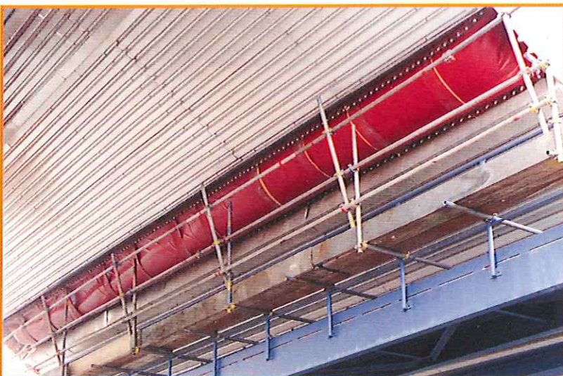
Multi-layer expansion-joint with insulation in a DeNOx plant for a coal fired power plant
